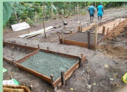
Nursery construction in progress: Crimping bed (in the front) and repotting bed (in the back)
