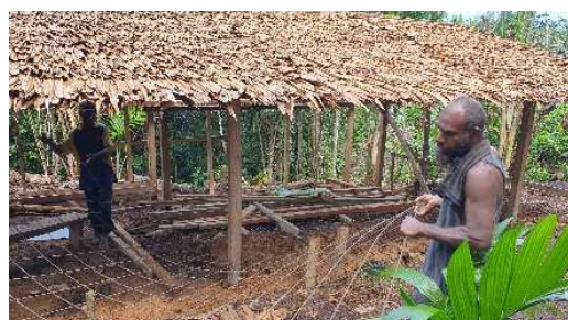
Concrete mesh wire for cement slab
