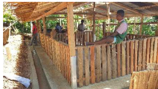
Drainage and partitions of pig stable
